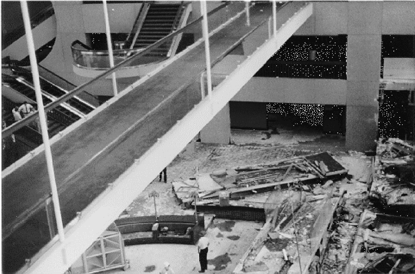
Figure 4: Collapsed walkways and 3 rd floor still hanging [6]
